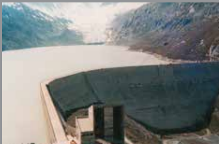
Grimsel Area Dam System, Switzerland
