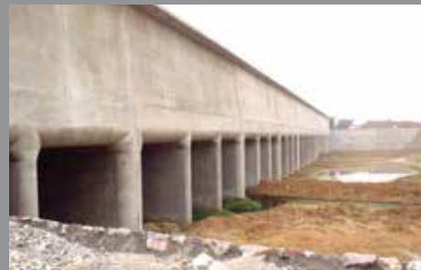
South-North Water Transfer Project, China
