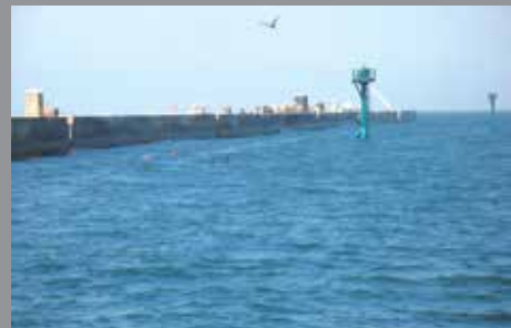
Sempra Energy Breakwater, Mexico
