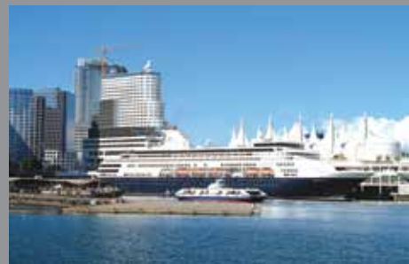
Vancouver SeaBus Floating Docks, Canada
