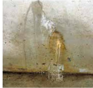
Leaking Joints
