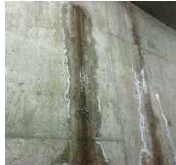
Leaking Joints
